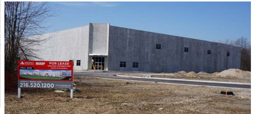
3620 Mallad Run High Bay Distribution For Lease
